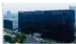
Hangzhou Production Base
